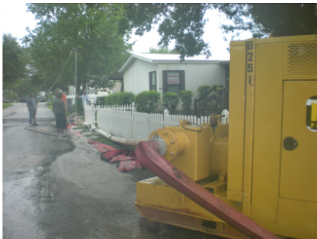
The City's Contractors work, even in the rain.
