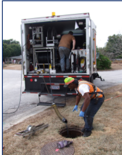
Lined sewers are televised to ensure a job is done correctly.
