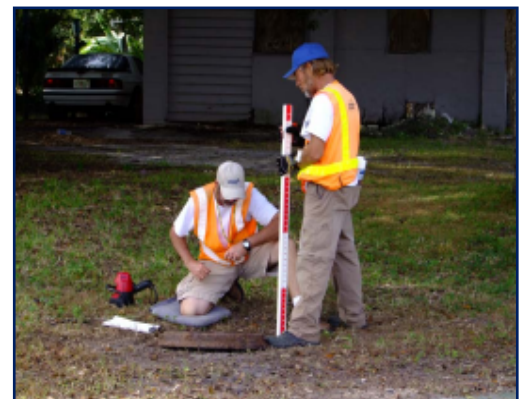
All sewer manholes are surveyed during the project so that the City of Sanford can create a hydraulic model of the
